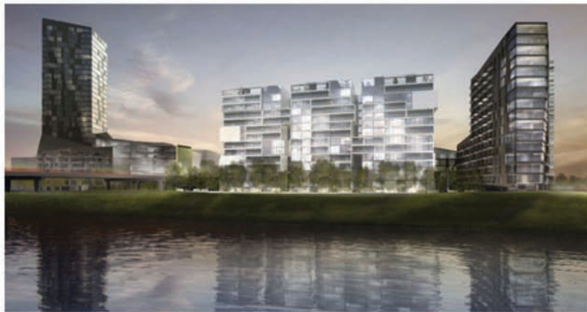
Phase two of River City is a 12-storey building divided into three mini-towers, connected by glass passageways.
